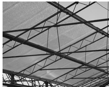
Fig. 7b. Detail of the roof construction of the wide span greenhouse in Assendelft.
