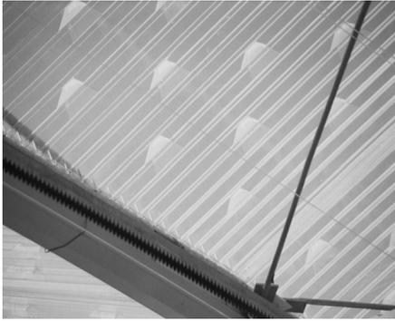
Fig. 5a. Vacuum formed ZigZag sheets with spacers in triangle shape between the inner and outer layer.
