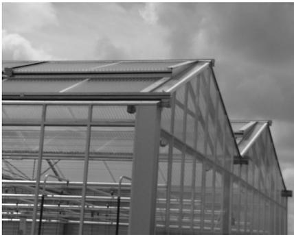
Fig. 6a. First greenhouse with Extruded zigzag sheets: Lexan<sup>®</sup> Zig Zag<sup>™</sup> in Elst (Netherlands).
